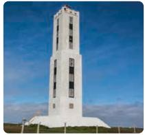
Built in 1938-1939, the Knarrarósviti lighthouse was the first one in Iceland to be built out of reinforced concrete
