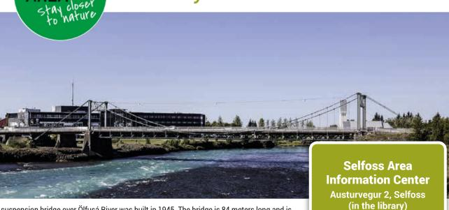
A suspension bridge over Ölfusá River was built in 1945. The bridge is 84 meters long and is in the town Selfoss
